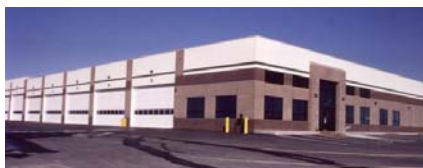
KCI Equipment Storage Building
