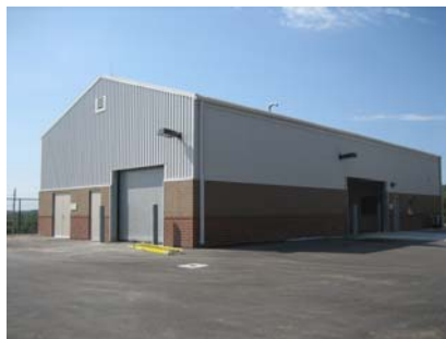
Storage / Maintenance Building Leavenworth
